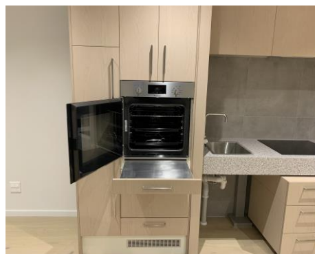
Images: The Lanes, Mermaid Waters Qld. Kitchen modifications made to facilitate room to roll under a height-adjustable benchtop, with oven modified for seated use. Toilet adjustable left-to-right on the wall to facilitate different tenants requirements.
